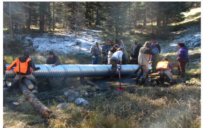
Right: Installation of the barrier culvert below pond four
